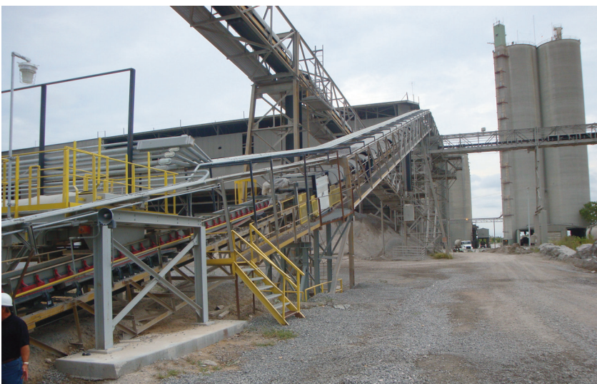
Figure 4. Before the upgrade, 550 ft long reclaim tunnel conveyor, which elevates material 138 ft at 400 tph, could not restart under full load.
