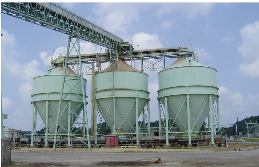
Figure 7. Single drive on reversing conveyor above woodchip bins slipped during winter weather due to stiff belt, prior to conversion to dual 15 hp. drives (one at each end).
