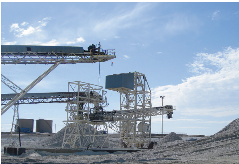
Figure 6. Radial stacker disrupted mine production due to belt slippage on 30 year old 100 hp. tail drive during rainy conditions
